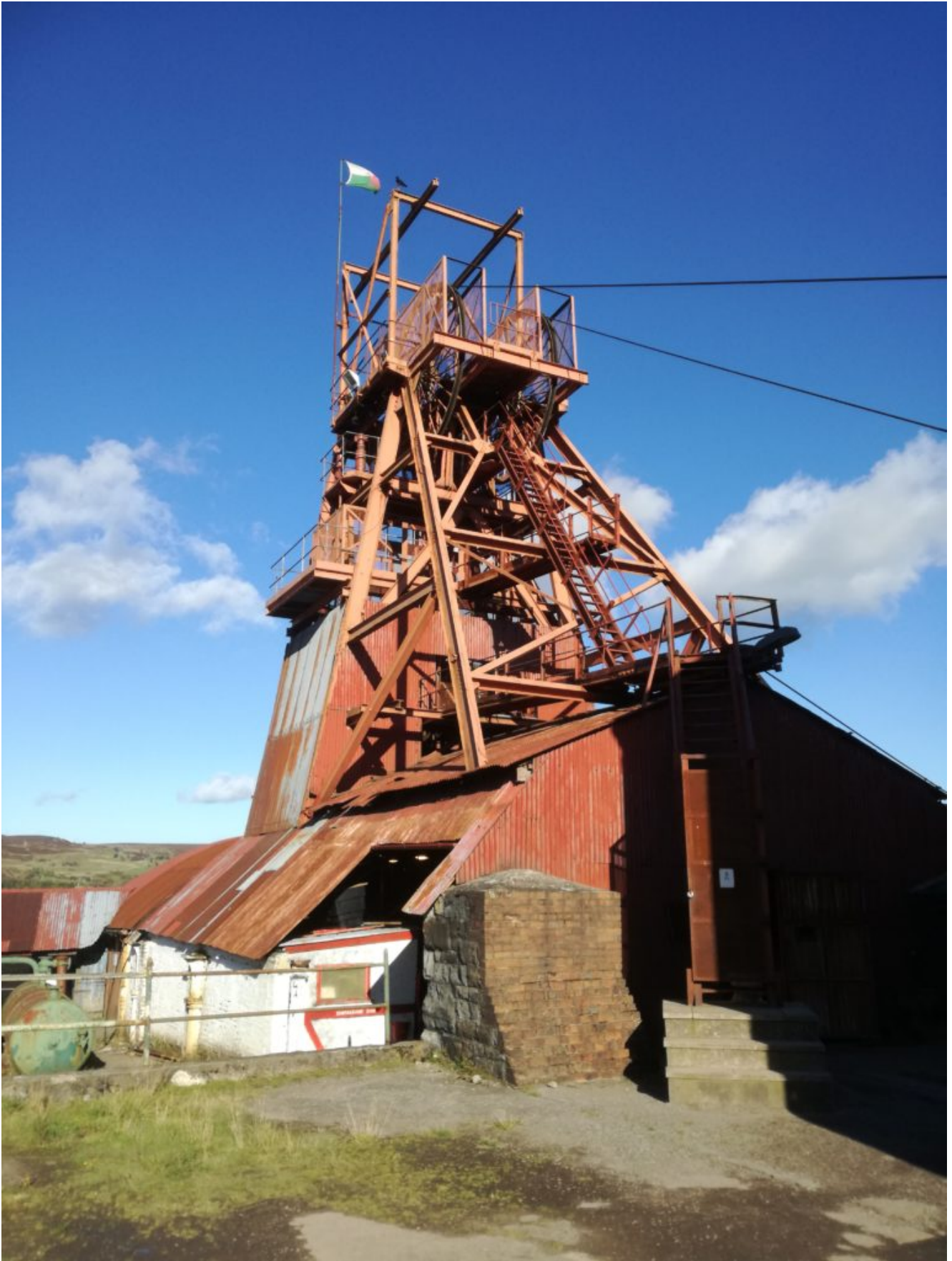
An award-winning national museum that still retains many features of its former life as a coal mine, standing high on the heather-clad moors of Blaenafon, the tunnels and buildings
